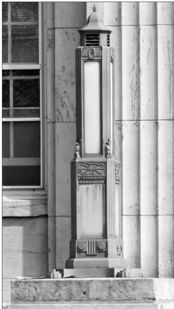
Fantastical light towers sculpted in cast aluminum rise like miniature skyscrapers on either side of the entrance. Like the building itself, they combine classical details in a modernistic form. Note the little cupola tops that mimic the large copper cupola that tops the building.
