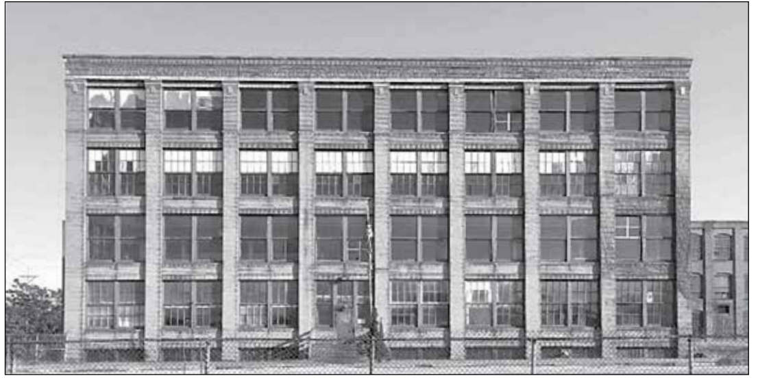
The "O" Building of the Annevar complex, which dates to 1914, demonstrates the simple, but elegant proportions that resulted from the desire to create a large, well-lighted interior in a simple straightforward fashion.
