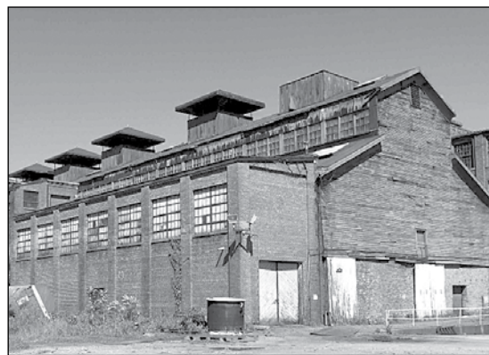
One of two great dye houses at the Annevar complex showing its long row of monitor windows and five great ventilators. The end wall was never finished, presumably because the company expected a further expansion.
